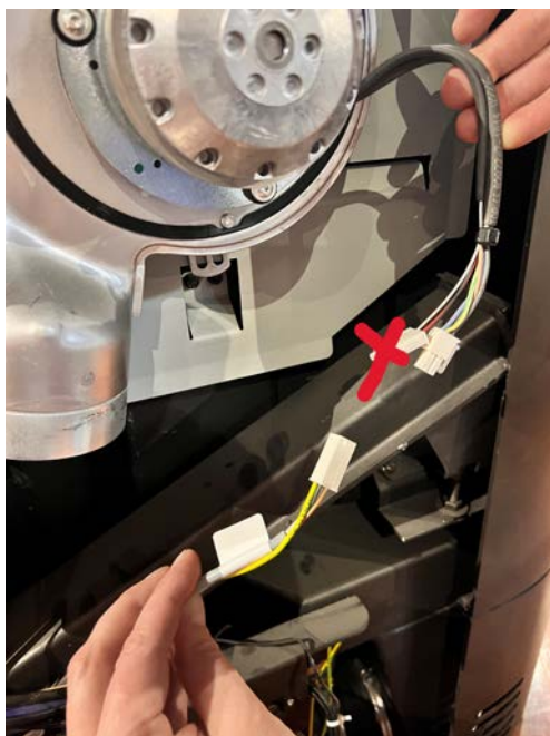
Fig. 23: Connecting the cables
