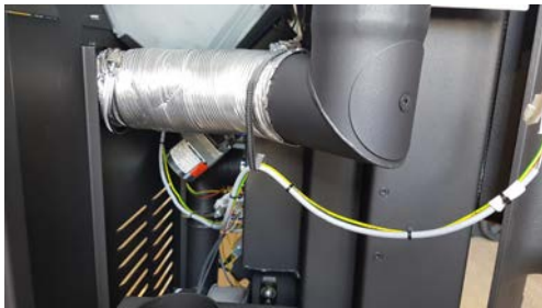
Fig. 78: Attach aluminium flexible hose.
