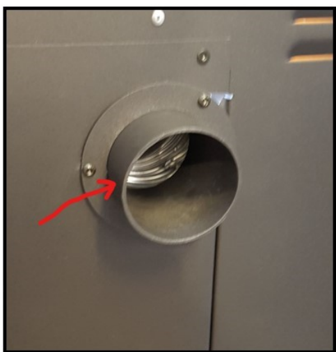
Fig. 89: Mounting the double connection bracket
